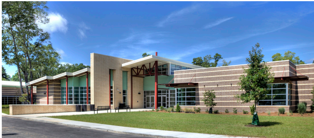
View of Front Entry/Auto Drop-Off
